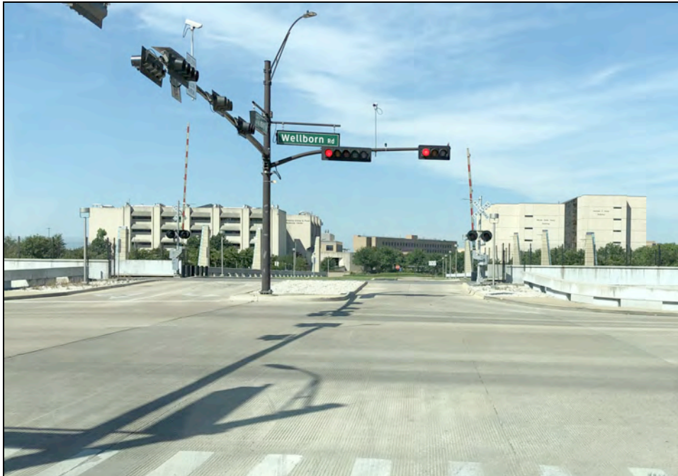
Westbound Old Main Drive DOT No. 743211Y
