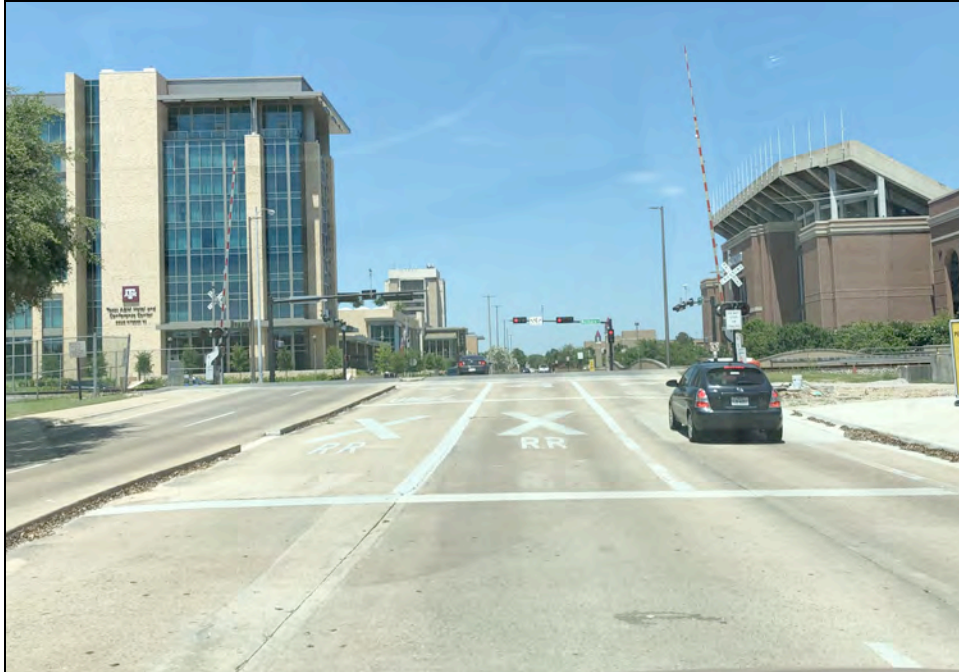
Eastbound John Kimbrough Boulevard DOT No. 743212F
